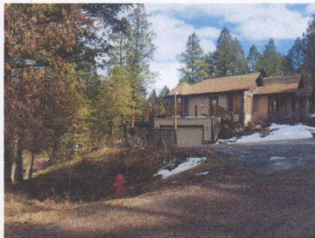
Figure 3: Fire Hydrant Location
